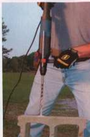
Masonry bits feature a chisel-like tungsten carbide tip and are often used with a pumping action to pull chipped material out of the hole.
