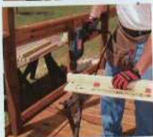
Adjustable pilot bits pre-drill screw holes to prevent splitting wood. They can also countersink screw heads flush with the wood surface.
